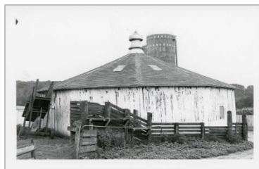
Polygonal Barn (no longer in existence) Source: 1986 NRHP nomination
